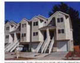
Inappropriate: Entry doors too high above street level.
