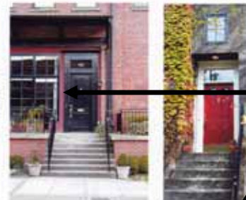
Appropriate: Recessed entry and high quality door and hardware set comfortably above the sidewalk.
