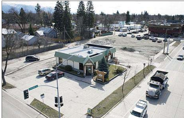
Several buildings remain at the Block 46 redevelopment site, including Whitefish Title Services and several homes along Kalispell Avenue, back of photo. Photo by gravityshots.com
